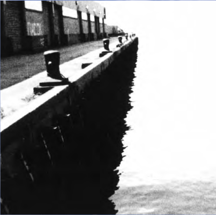
13W Trapezoidal Northeast Terminal Pier, New York, NY
